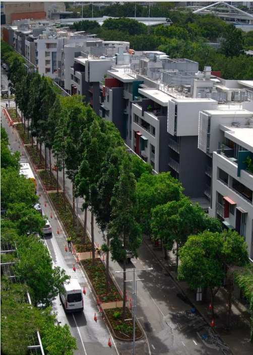
Grey Street Improvement works – Stage 1. (Photo courtesy of: I. Hume local South Bank resident).
